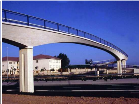
Image 3-15. Bridge post-tensioned on site with variable edge.
