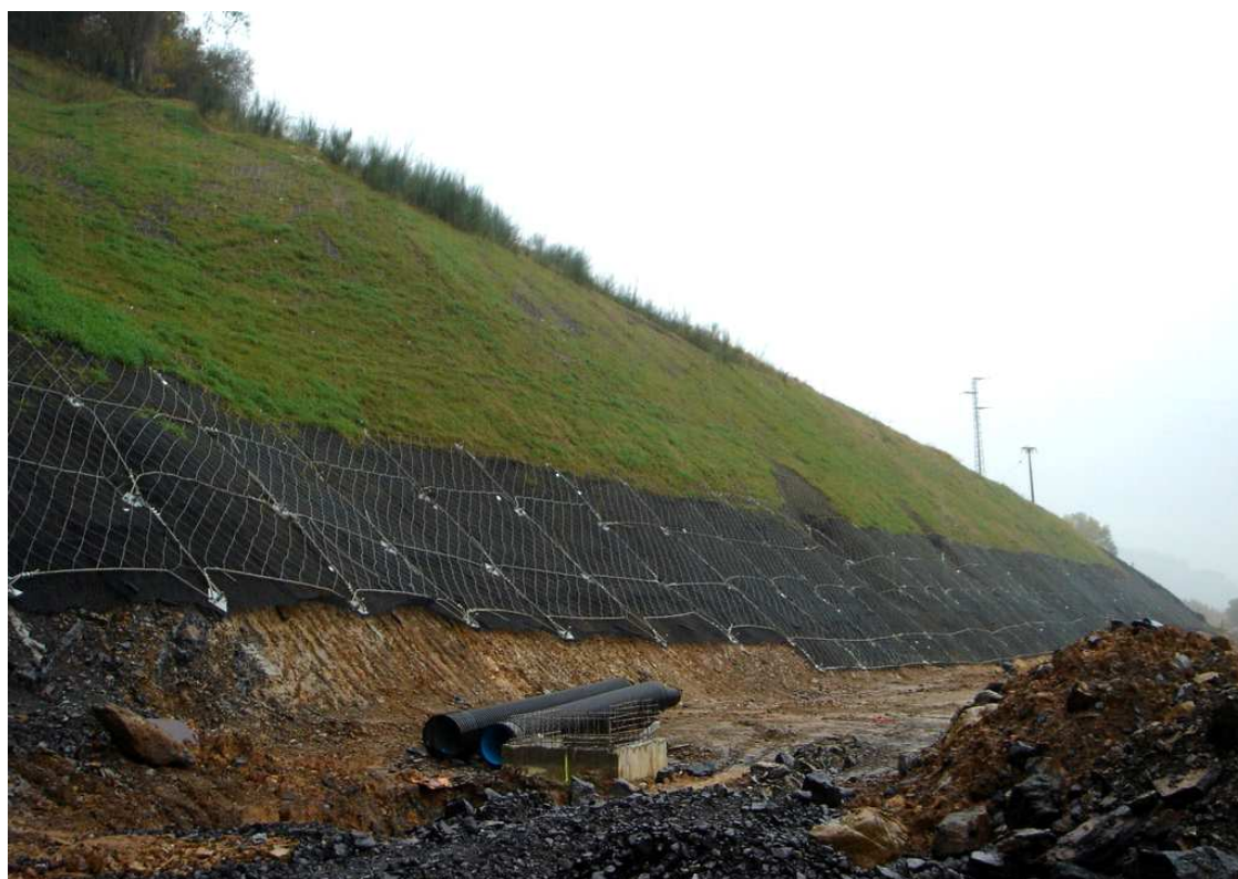
Image 3-27. Detail of geotechnical correction in slope.
