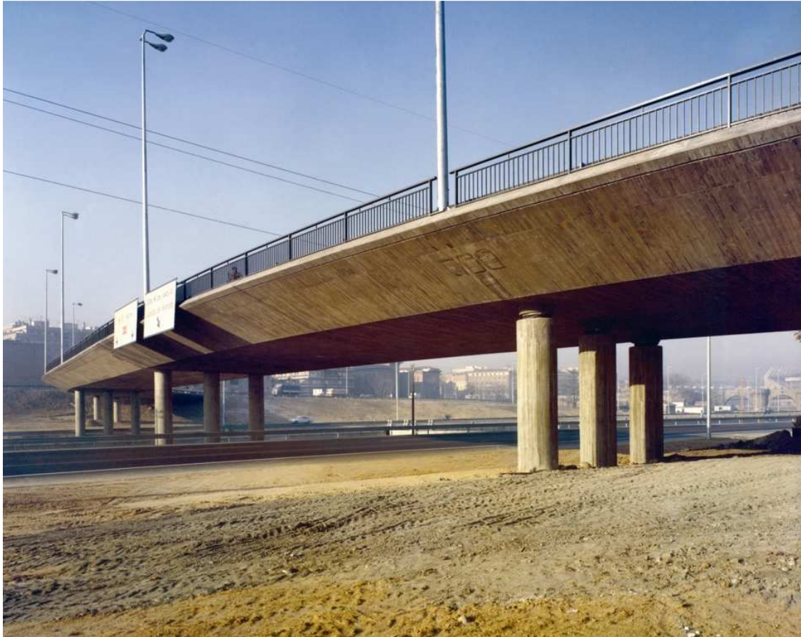
Image 3-14. Bridge post-tensioned on site with invariable edge.
