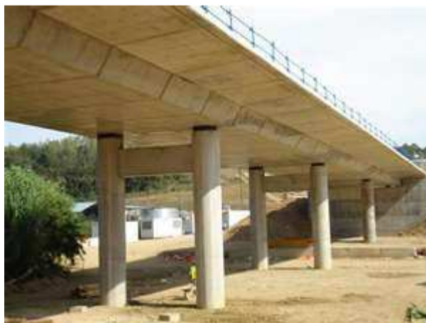
Image 3-10. Example of slab bridge made with circular voids.
